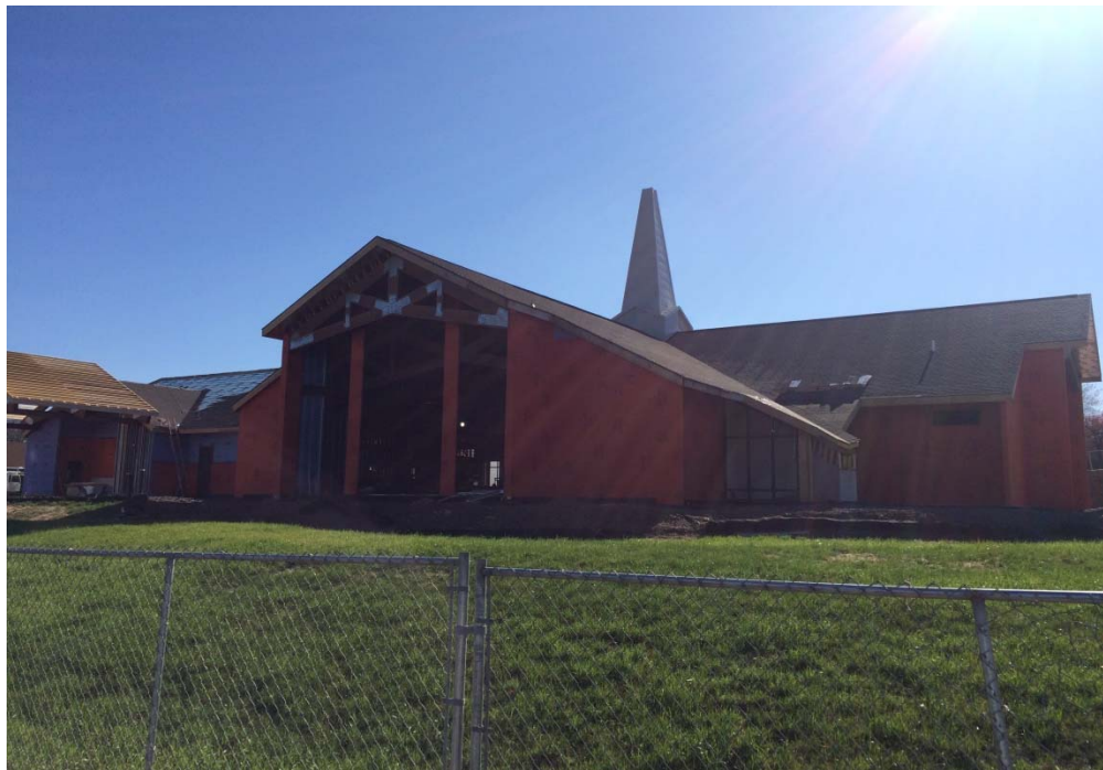
Looking north east picture taken from Route 309
