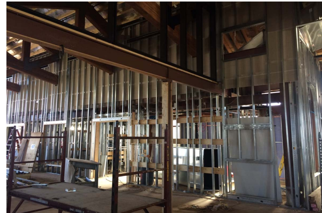
Drywall being installed in mezzanines as required.
