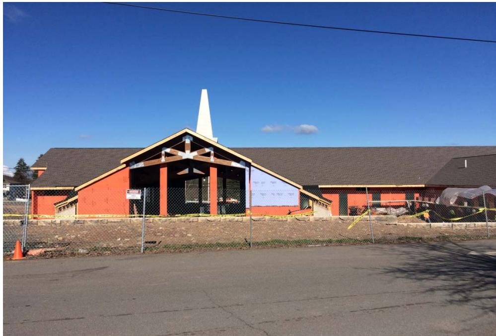
Looking West from access road.
